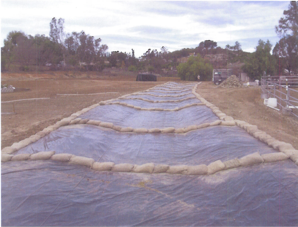
Visqueen channel constructed by City of Poway contractor
