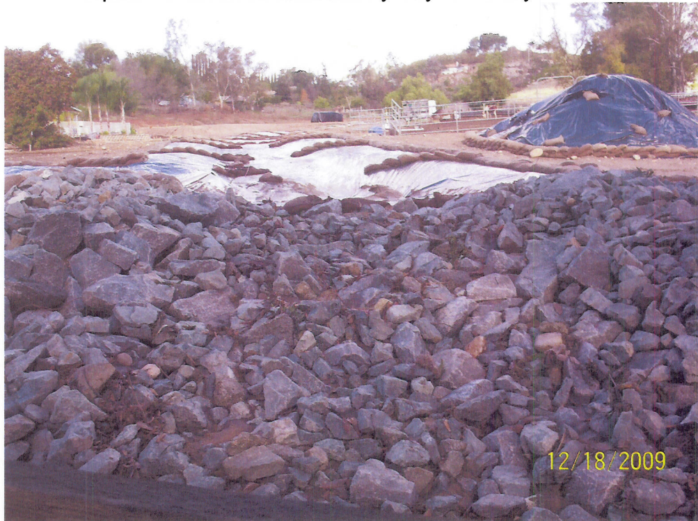
Riprap energy dissipation at southern edge of property
